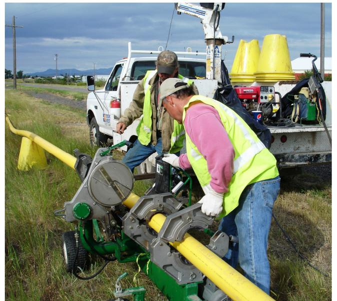
PA11 — like PA12 — is a nylon material; however, PA12 contains an extra carbon atom that has a minimal effect on chemical resistance, performance, and strength. As a result, there are no significant differences in the overall strength and long-term performance for PA12 as compared to PA11. The primary advantage for the use of PA12 as compared to PA11 is that, while there is only one current supplier of PA11 materials, PA12 is available through four resin suppliers.
