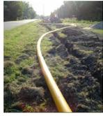
In this program, researchers evaluated the use of Polyamide 12 (PA12) polyethylene pipe for high-pressure gas-distribution applications. The introduction of new plastic materials — such as PA12 piping (designed to operate at pressures between 100 to 300 psig) — will allow utilities to use plastic pipe at higher pressures and temperatures than possible with current plastic materials.
