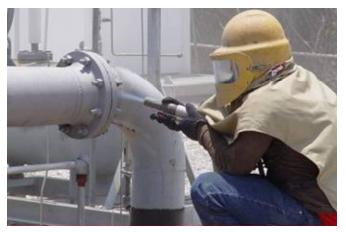
Surface preparation for tests of flame powder system.
